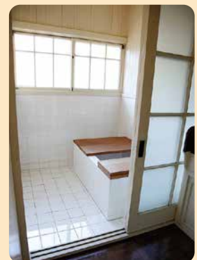
House of Okawa in Den'enchofu Built : 1925 6
