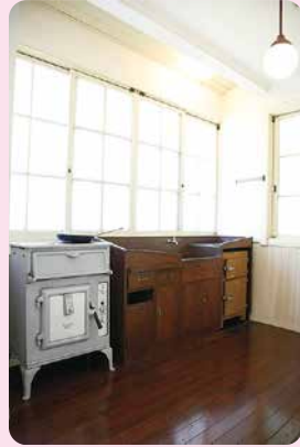
House of Okawa in Den'enchofu Built : 1925 3
